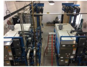
The water treatment plant was designed to be able to produce 980m<sup>3</sup>/day; in 2017 the plant produced a total of 182,587m<sup>3</sup> of treated water to the Town of Mahone Bay.
